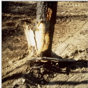
Tree injured during regrading. Photo credit: Joseph OBrien, USDA Forest Service, Bugwood.org
