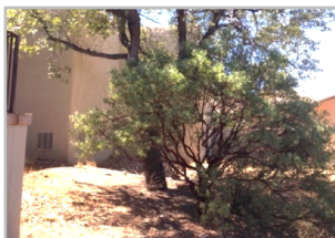
Large tree was vulnerable to wildfire due to shrub/understory
