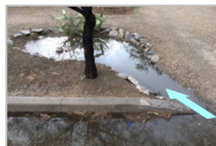
Curb cut harvests street runoff
