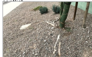
Tree on slope has exposed roots due to erosion and needs heavy staking for stability
