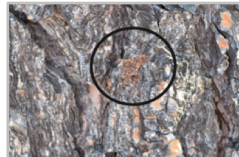
Reddish brown boring dust
