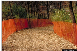
Fencing marks access around trees during construction, and woodchips reduce compaction over roots. Photo credit: Paul Bachi, University of Kentucky Research and Education Center, Bugwood.org
