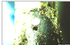
Round exit hole 0.4 inch
