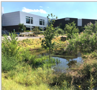
Large-scale green stormwater infrastructure. Photo credit: MRWM Landscape Architects
