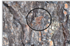
Reddish brown boring dust
