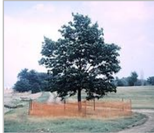
Fencing protecting tree during construction. Photo credit: Peter Bedker, Bugwood.org
