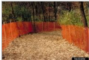
Fencing marks access around trees during construction, and woodchips reduce compaction over roots. Photo credit: Paul Bachi, University of Kentucky Research and Education Center, Bugwood.org
